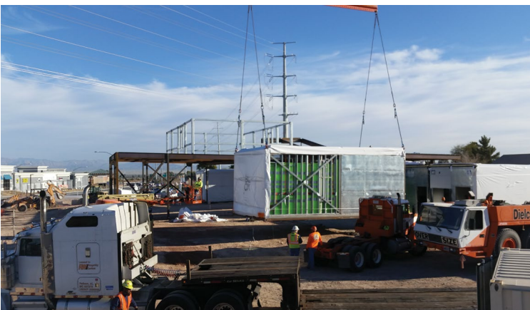
Photo of BLOX Built construction site
